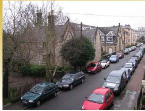
:: York Road – spring 2009 /km
