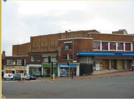
:: Cinema site / Ritz Building - 2009 /db
