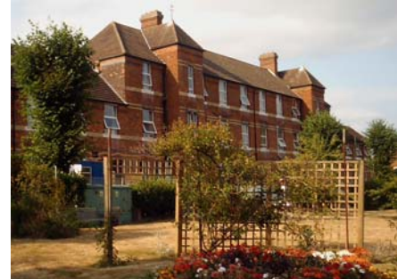
A view of Pembury Hospital
