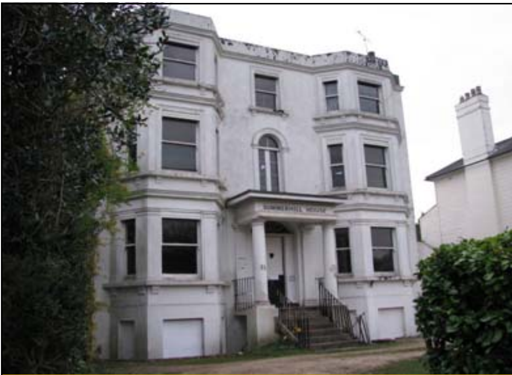
Summerhill House, 73 Inner London Road revisited – db / April 2008
