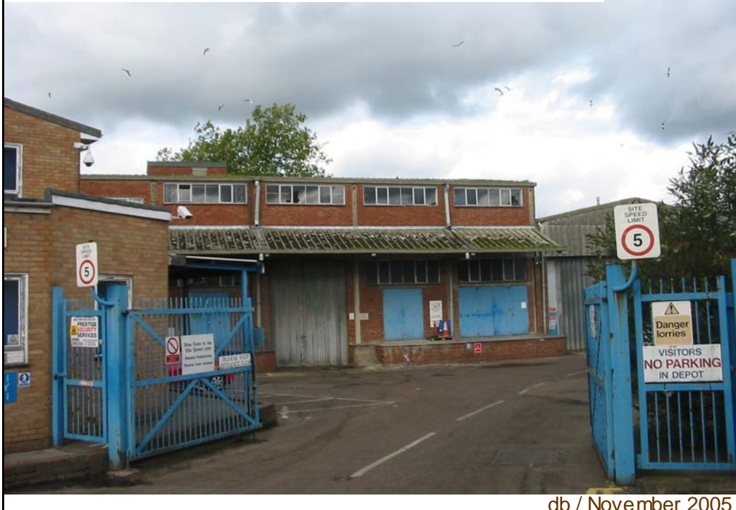
Medway Depot – Corner St James Road
