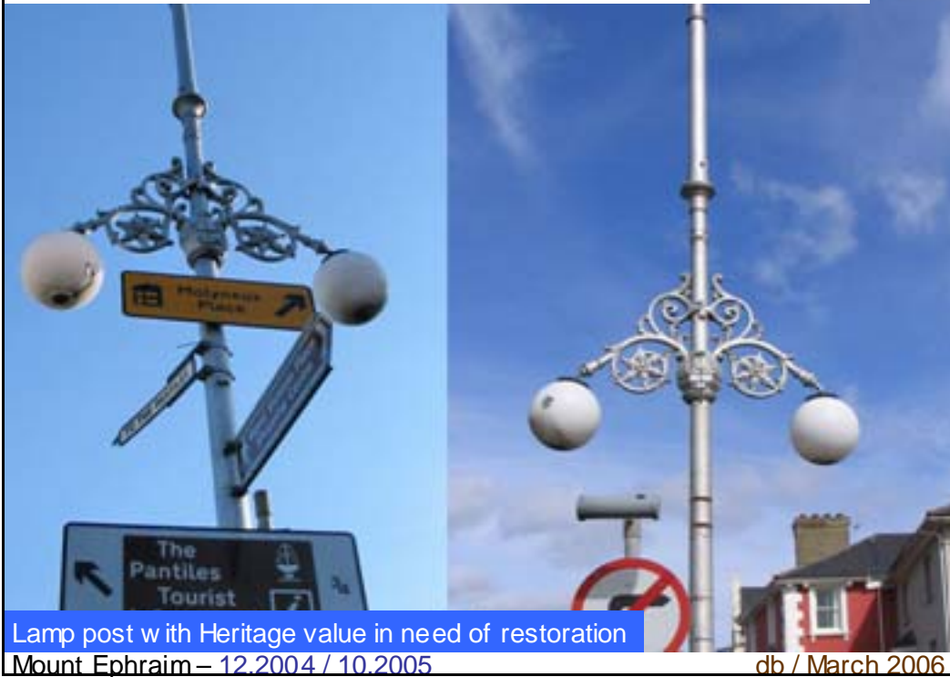
KHS 04.2006: 16. Before and after shot of de-cluttered lighting column
