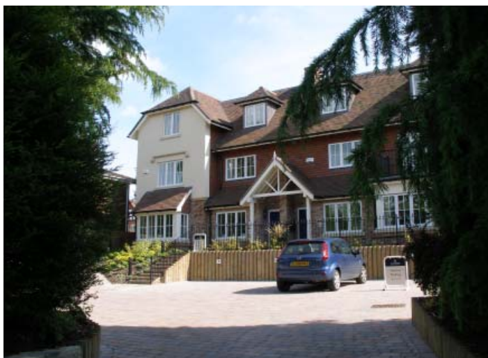
A recent garden development in Forest Road
