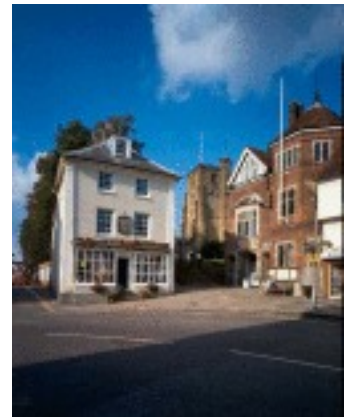
Picture 5 Vestry Hall, Cranbrook
