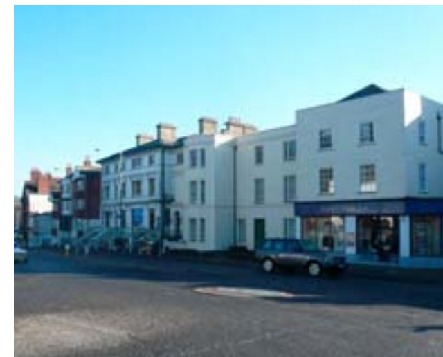
The London Road frontage
