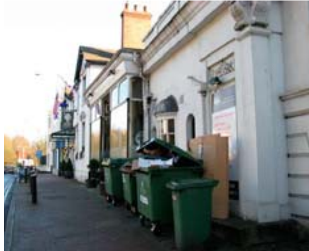
Pavement clutter on London Road
