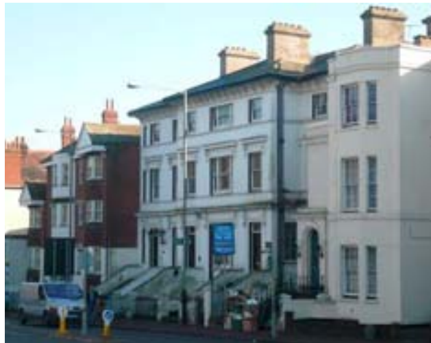
Maintenance issues - London Road
