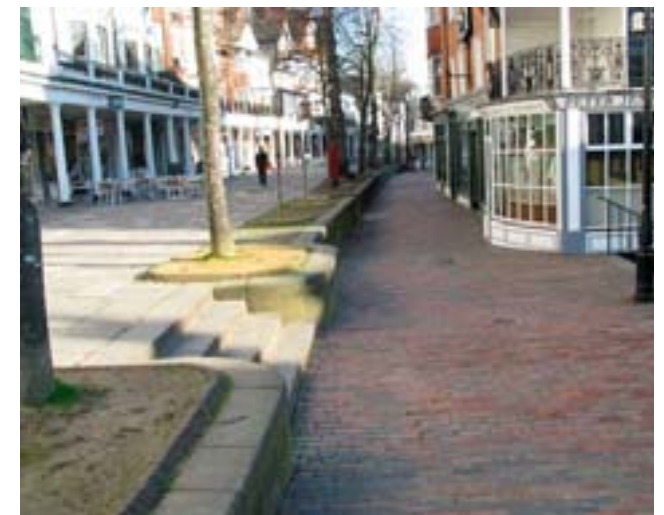
The listed paving and change in levels
