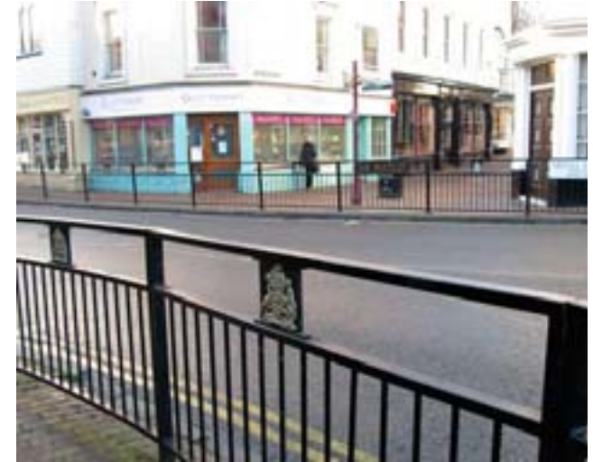
Guardrails blocking natural desire line - Nevill Street
