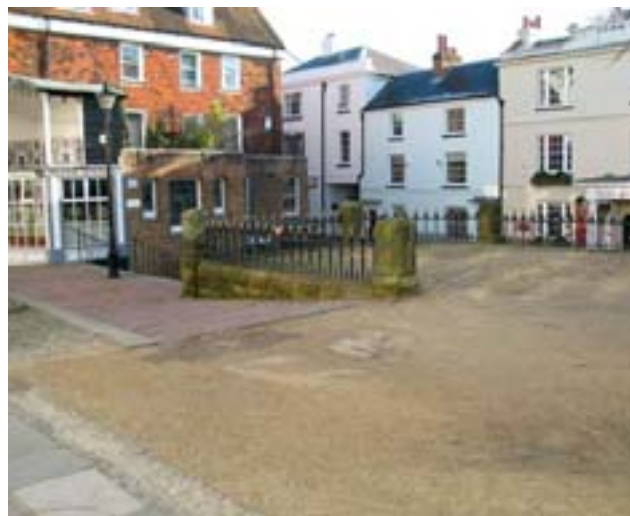
Deterioration of the public realm
